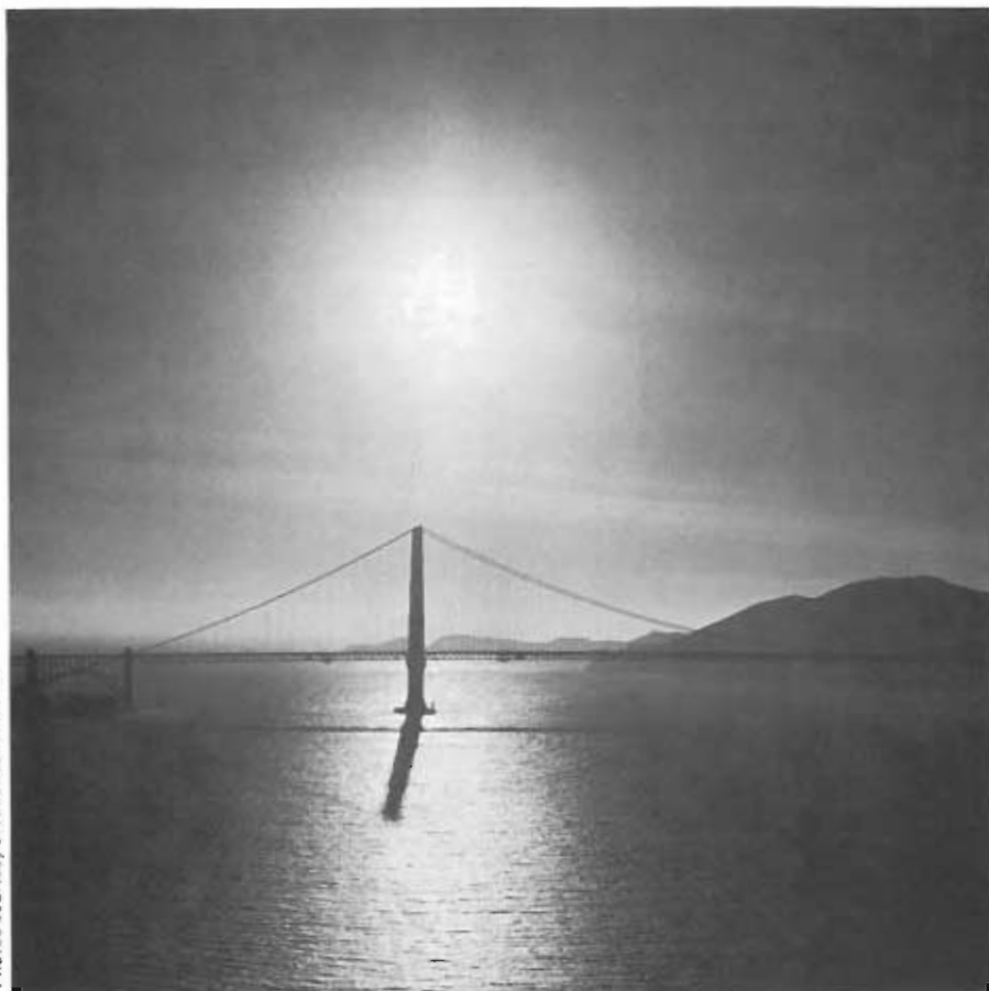
The Golden Gate Bridge at Dusk.
